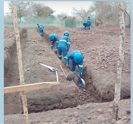
Foundation preparation in Chicuacha Primary School construction, in Chibabava, October.
