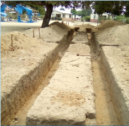
Foundation preparation in Chipinde Primary School construction, in Dondo, October 2020.
