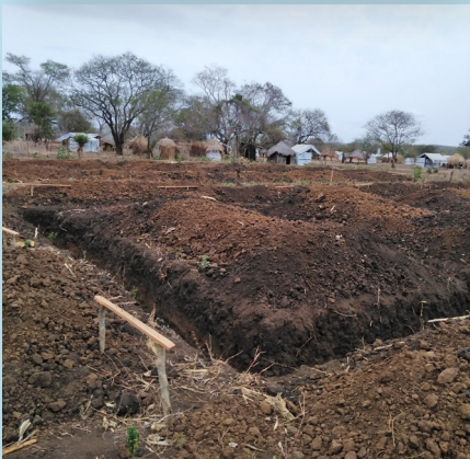
Demarcation of the site in Muconja Primary School, in Chibabava.
