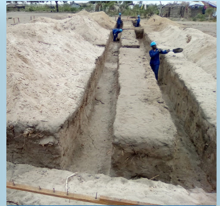
Foundation preparation in Mutua Primary School construction, in Dondo, October 2020.
