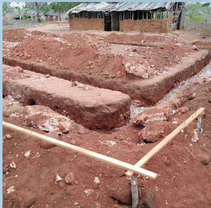
Demarcation of the site in Heua Primary School, in Chibabava, October.
